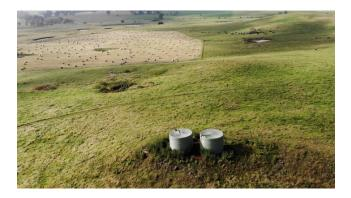
Figure 4: Tanks located on hill so that water can gravitate to troughs, this can eliminate the need for extra pumps
